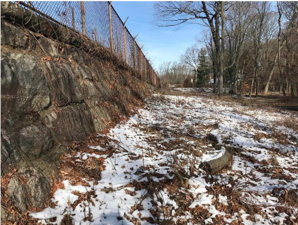
Photo No. 10: View of masonry dam left side of the spillway.
