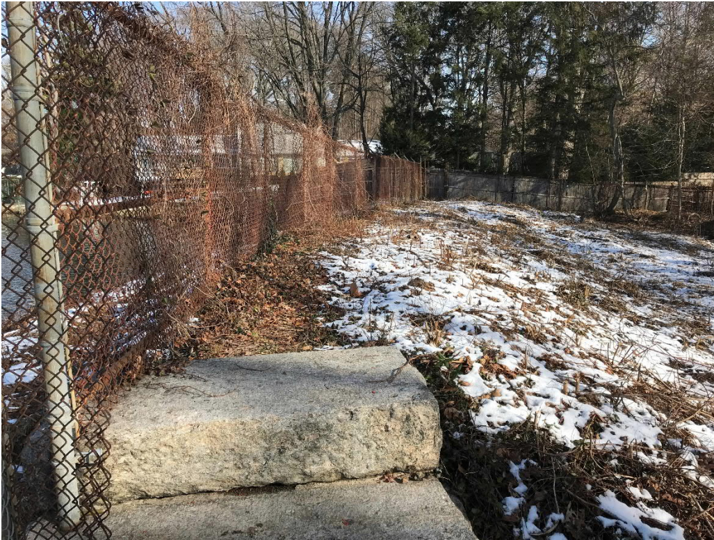
Photo No. 13: Masonry dam abutment to left earthen dike.
