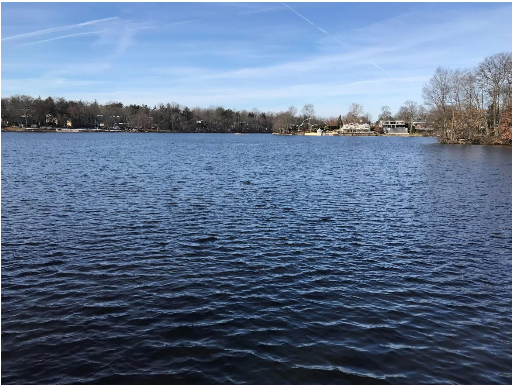
Photo No. 16: View of the reservoir from the masonry dam left of the primary spillway.
