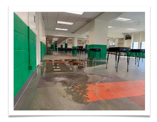
The cafeteria suffered serious damage and will be unusable for an extended period of time. The concrete slab underneath the floor is sinking. The flooring – installed two years ago – will need to be removed and a new concrete floor will need to be poured.
