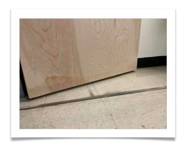
A brand new door has a visible waterline. The door will need to be replaced.
